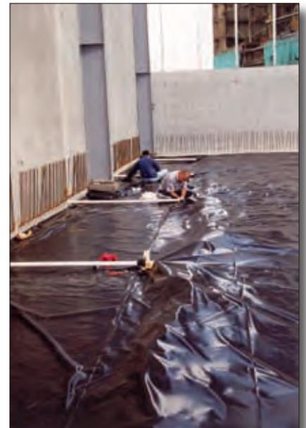
Then total area of approximately 4300 m<sup>2</sup> was covered with 8 panels of Permaliner prefabricated in the factory under ideal quality control conditions. These panels were joined on-site with Vulcaneal (1 mm rayon reinforced isobutylene isoprene) moisture and vapour resistant double sided tape and installed by Permathene.
