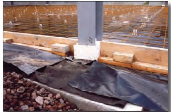
Permaliner FPP (Flexible Polypropylene) .5 mm geomembrane was specified to be placed between the top of the subbase course and the concrete slab. Permaliner geomembrane offers excellent gas barrier characteristics and is resistant to most chemicals. In landfill applications, the principal gases generated are methane & carbon dioxide.
