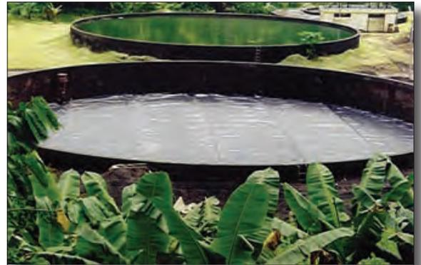
For rehabilitation of the filters, it was suggested by engineers to remove sand and wash it and prevent further infiltration of fine silt material into the lower gravel layers. To achieve this, Syntex GHS 35/35 high strength woven geotextile was recommended to be placed on top of the gravel layer because of its high strength and superior hydraulic properties.
