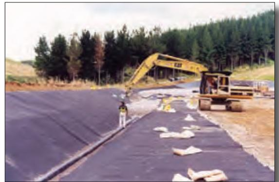
Syntex GNP E1 has been specifically designed for use in landfill or waste disposal facilities. United States Environmental Protection Agency (EPA) 9090 accelerated testing performed on this product has demonstrated an excellent chemical compatibility with landfill leachate. It is highly resistant to puncture, impact and abrasion, which greatly reduces the potential damage from sharp objects during and long after the construction process.
