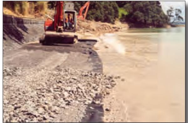
The contractor selected Syntex GHS 70/70 (70 kN x 70 kN) Woven High Strength Geotextiles based upon its excellent performance on similar projects.
