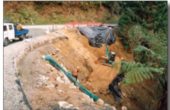
After thorough discussion with the Contractors, Syntex GHS 35/35 (35 kN x 35 kN) and GHS 70/70 (70 kN x 70 kN) High Strength Woven Geotextiles were approved for use in the construction of the Mechanical Stabilised Earth (MSE) wall.
