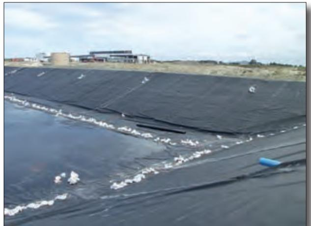
In addition to the fact that no excavating was allowed, the wetland terrain made this project exceptionally challenging, During preparation of the site, underground drains pumped water from the area to be lined and bund walls were formed. This made the site inaccessible to vehicles and a road had to be built to allow access to the area and enable installation of the liner to commence.
