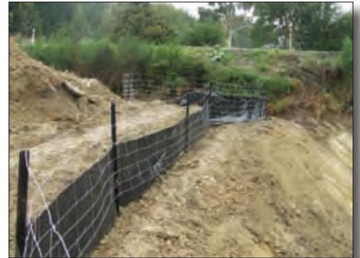
Ultra Violet stability is an important property of the Syntex silt fence used in this high exposure application. The high tensile strength of the fabric also ensures the continued performance of the fabric as sediment accumulates.
