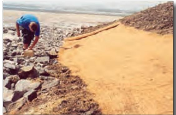
Landlok C2 is utilised to establish grassed waterways in low-flow drainage ditches and channels and along stream banks where moderate velocity intermittent flows may occur.
