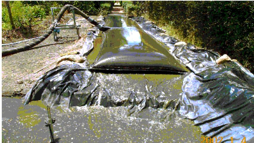
**Photograph 3. Geotextile tube being dewatered.**
