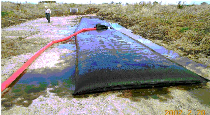
**Photograph 2. Filling operation of the geotextile tube.**
