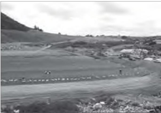
The GCL was installed before the HDPE sheets were lapped and joined using a twin track, hot wedge-welding system. The double seam gives extra security against leakage and also provides a sealed tube between the two seams that was finally pressure tested to ensure that the adequate seal was achieved. The fusion welds were tested for peel and shear strength using a field tensiometer. All extrusion welds were spark tested to check their integrity.
