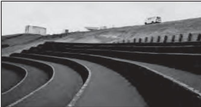
**L**andlok TRM 450 turf reinforcement mat was used in this project to enhance the natural ability of plants to protect soil from erosion and improve the beauty of this regional park. By using a flexible three dimensional turf reinforcement system on a slope or a bank, seed and soil is retained and seed
