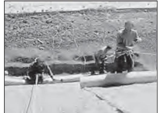
**Vercan** Root Barrier: A textured high density polyethylene specially designed to confine tree roots. Easy to install by using a narrow width excavator and flexible to form any contour, Vercan Root Barrier is the simple long term solution to prevent cracked paths, roads, pipes and damage to other utilities.
