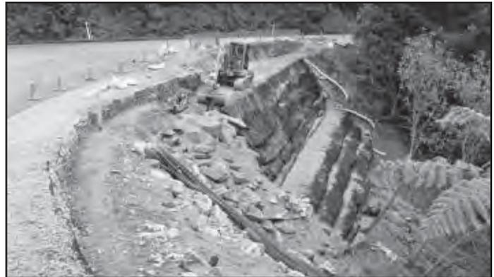
was laid over the compacted Onekaka Schist Sandy soil. This sequence was repeated until the wall reached its total height of 6m. Hydroseeding the wrapped face of the wall was suggested. Syntex is distributed by Permathene Ltd in the Pacific region and India.
