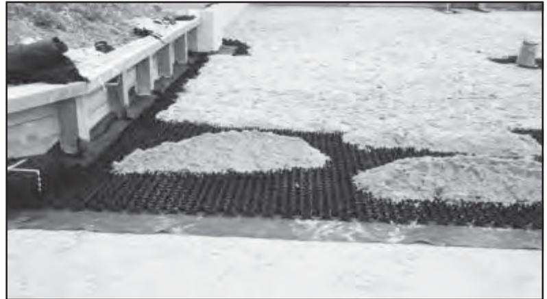
HDPE grid structure specially designed to stabilise and support turf, grass or decorative gravel. It allows the creation of stabilised and durable lush lawns, which add to the quality and beauty of the environment. Simple and economical to install, resistant to UV, acids, alkalis, extreme temperatures.
