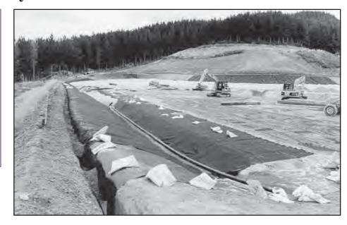
designed for use in landfill or waste disposal facilities. United States Environmental Protection Agency (EPA) 9090 accelerated testing performed on this product has demonstrated an excellent chemical compatibility with landfil leachate. It is highly resistant to puncture, impact and abrasion, which greatly reduces the potential damage from sharp objects during and long after the construction process.
