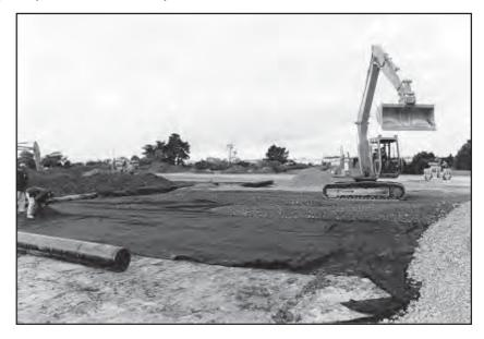
included hydraulic filling, construction of slab culverts, pipe culverts, retaining wall construction of road crust protection works consisting of stone pitching, gabions filled with stone boulders and placed over geotextiles as advised by Permathene Ltd.
