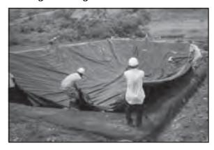
ermathene was involved with the designing of this project with Harris Consulting of Auckland. Based on available site soil data 750mu **Permaliner** FPA polypropylene and **Syntex** 1001 nonwoven geotextiles were specified for these backwash ponds. The lining was manufactured at the Permathene factory in Auckland as a single one piece membrane and transported to Fiji for installation.
