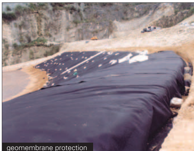
separation, stabilisation, drainage
