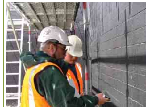
Permathene installation crew at former brownfield site, Abbots Way, Auckland, New Zealand (2006, 2007)
