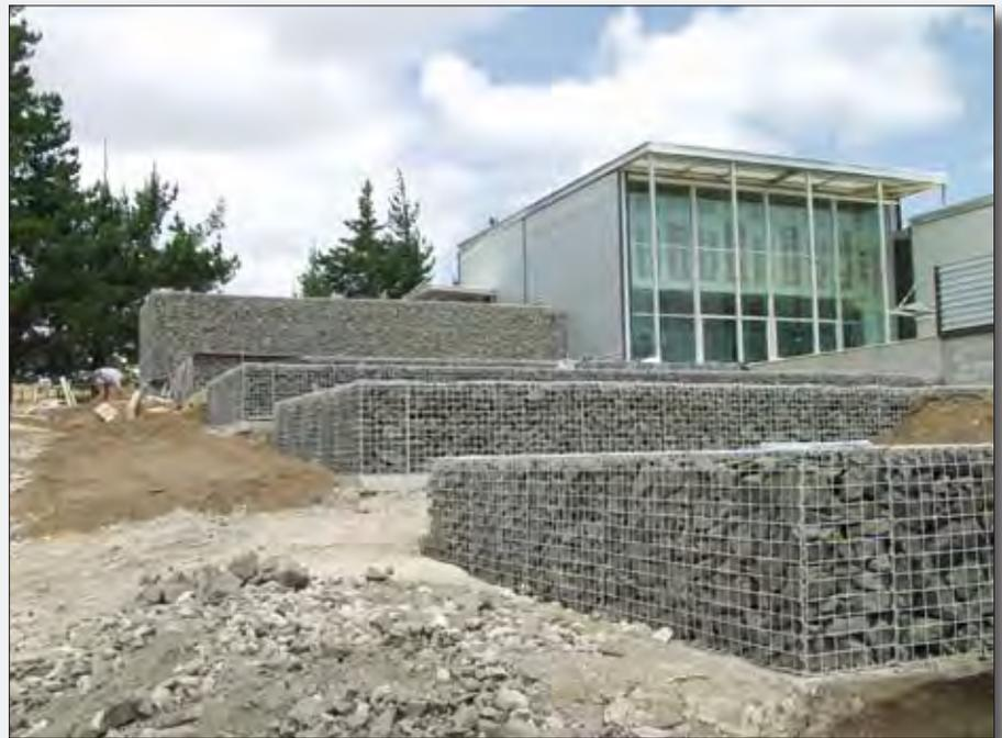
Gabions have the advantage as a hard armour system due to the fact that the rocks within the system dissipate energy of wave action, floods, etc. Silt and vegetation will eventually collect within the gabion wall forming an environmentally friendly and sound structure which is, for the most part, completely maintenance free. Installation is fast and easy and can be done using unskilled labour. Rocks can be found locally.
