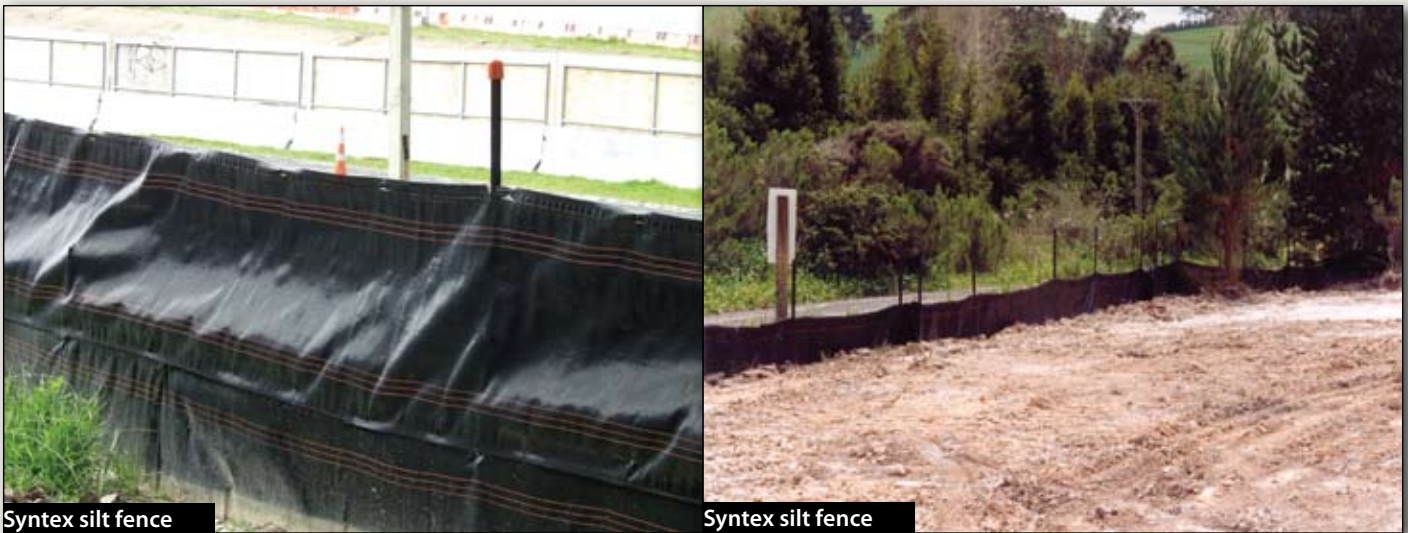
Syntex silt fence
